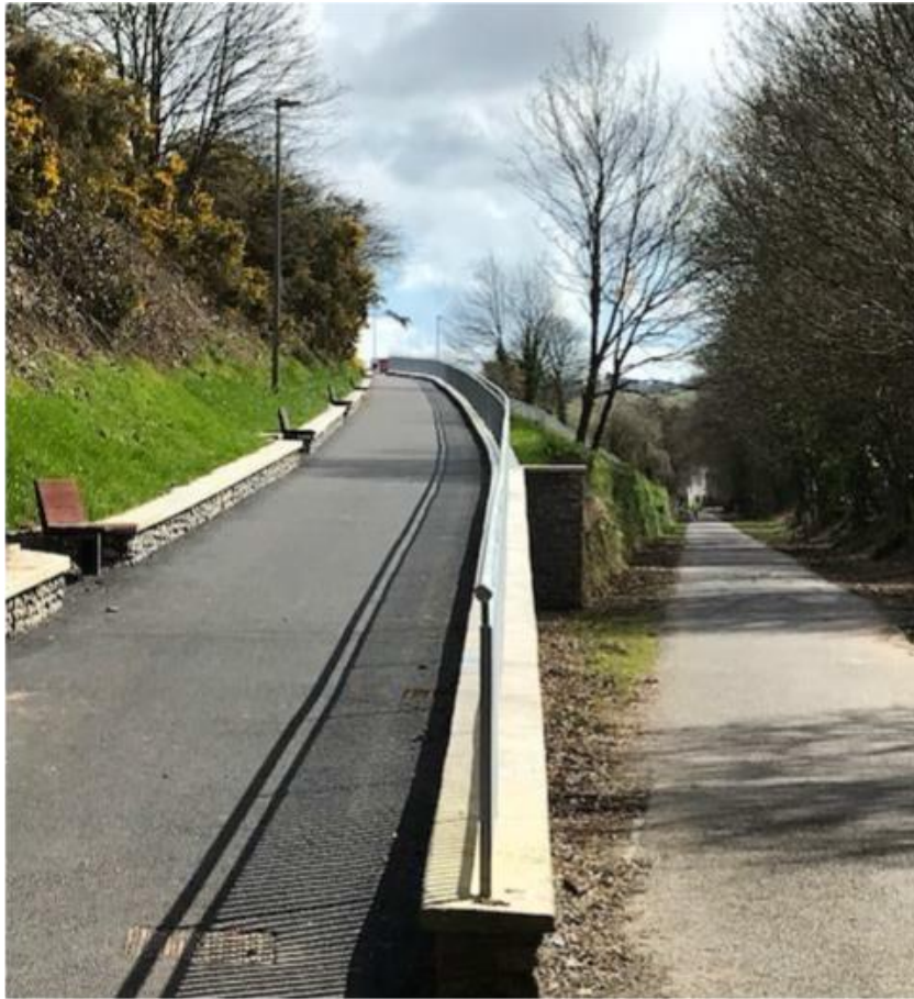
Figure 25 New Cycle Ramp access at junction of Mahon Link Road and St. Michael's Drive
