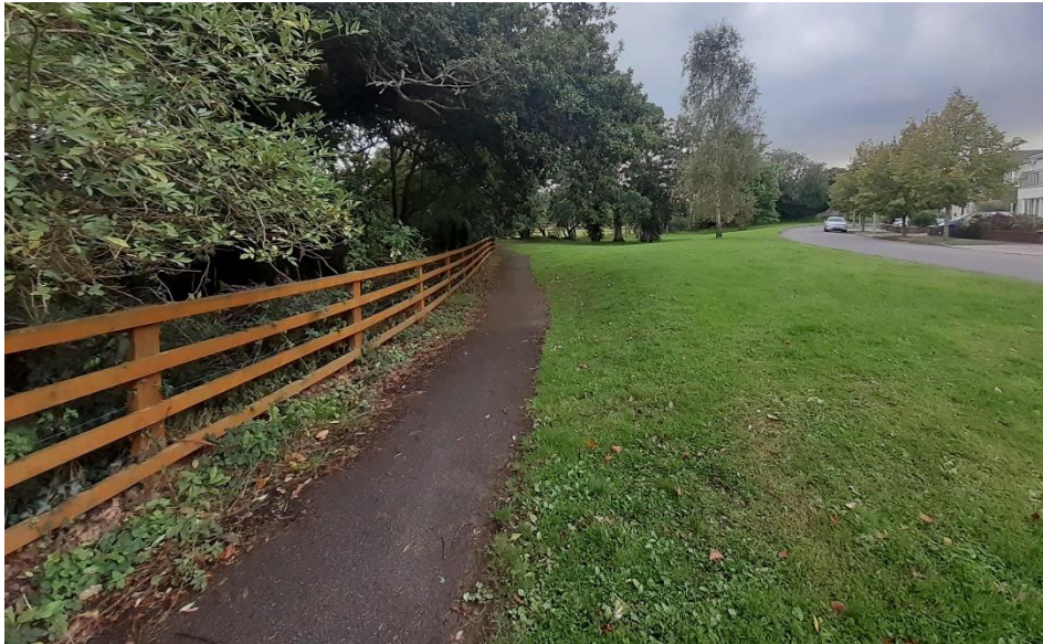
Figure 21 Footway at Joe McHugh Park Mahon
