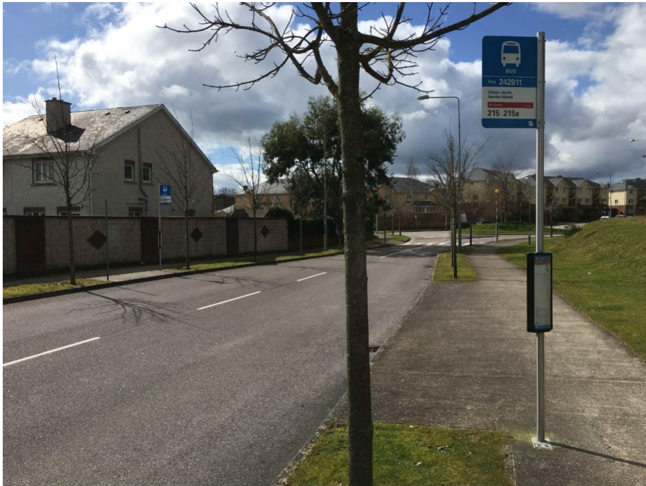
Figure 15 Existing Footpath facilities on Jacob's Island
