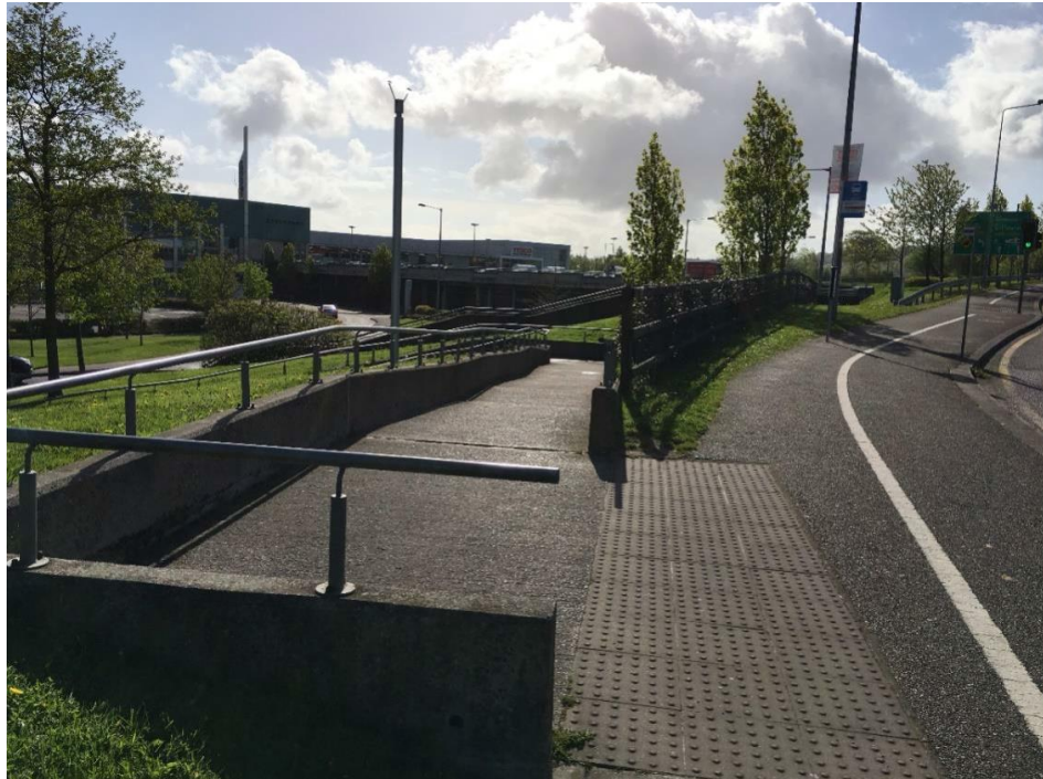
Figure 13 Pedestrian Accessibility to Mahon Point Shopping Centre from Mahon Link Road
