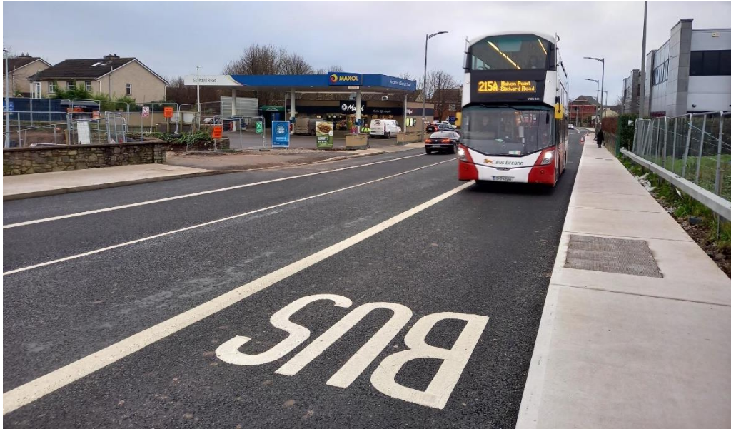
Figure 6 New bus lane on Skehard Road
