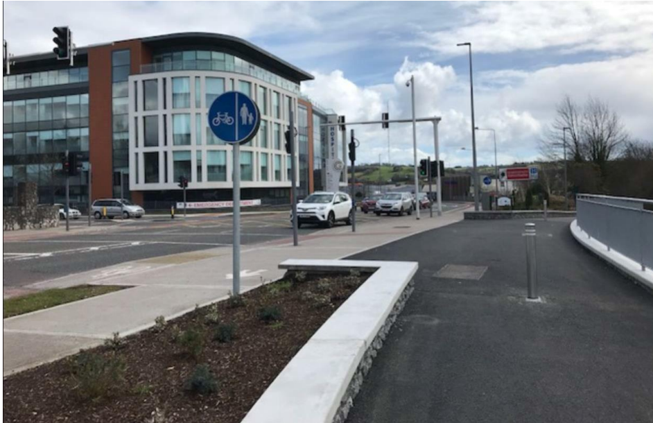
Figure 24 New Cycle Ramp access at junction of Mahon Link Road and St. Michael's Drive
